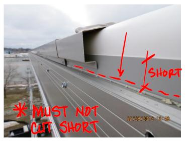
We recently had to deal with a water intrusion issue on the interior of a metal panel system due to the roofing being cut too short. Water got under the parapet, backed up, and went into the building.
