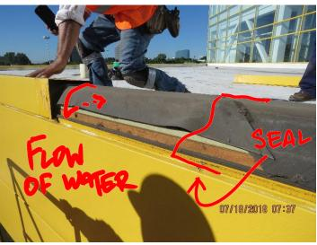
Roofing not cut or terminated properly, which allows water to get past the system and leak on the interior
